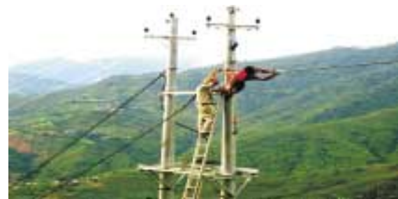
Line Erection in Dhankuta
