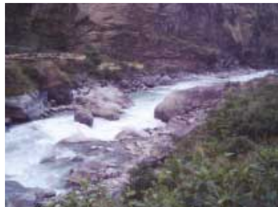
Upstream View of Upper Trishuli - 3A Headworks Site
