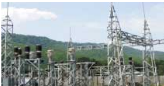
Substation Construction works in progress in Mukundapur
