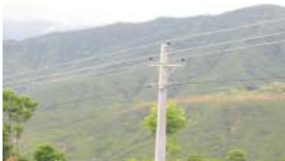
Line erection in Ilam
