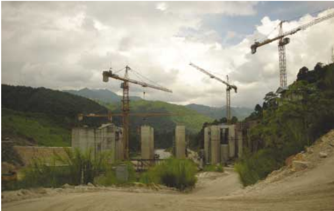
Upstream View of Diversion Weir -Middle Marsyangdi HEP
