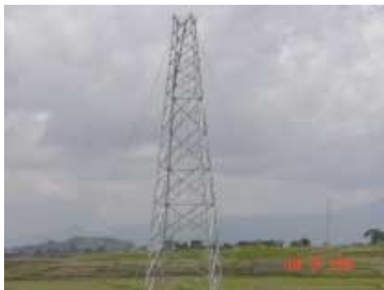
Tower Installation under Thankot-Chapagaon-Bhaktapur 132 kV Transmission Line
