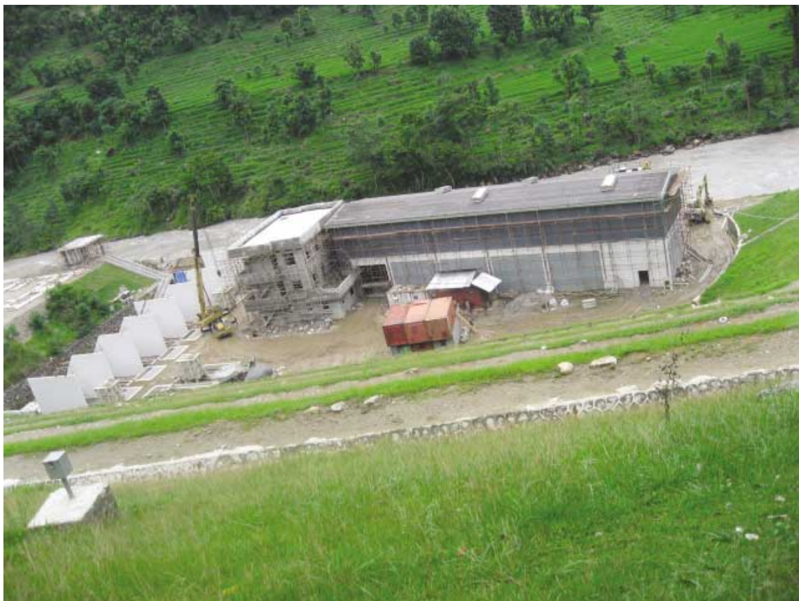
Middle Marsyangdi Power House nearing Completion
