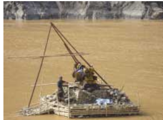
Drilling at Proposed Sunkoshi Diversion Headwork Site
