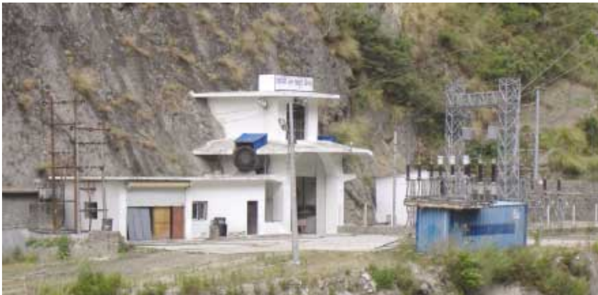
Switchyard and Adit to Powerhouse
