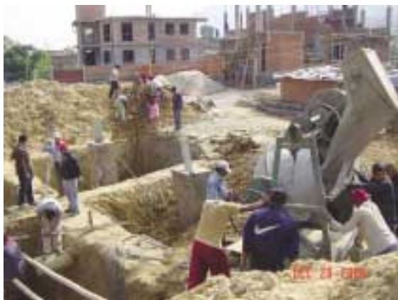
Constructing Chandranigahpur 132 kV Substation
