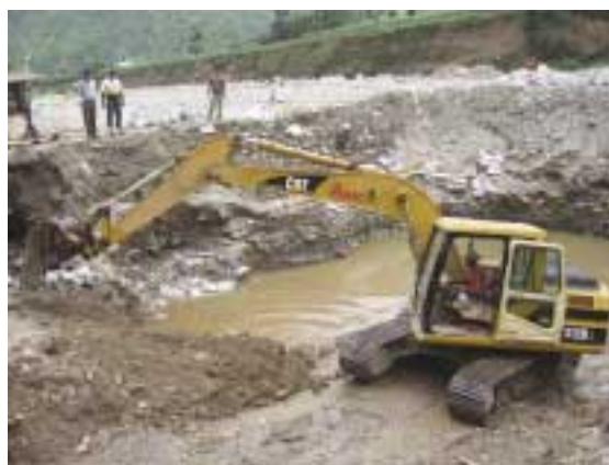
Bridge foundation work of Kulekhani - III HEP
