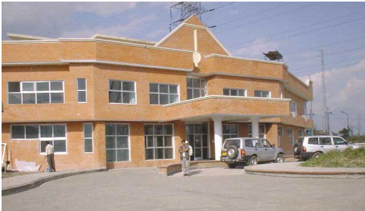
LDC Building at Siuchatar, Kathmandu
