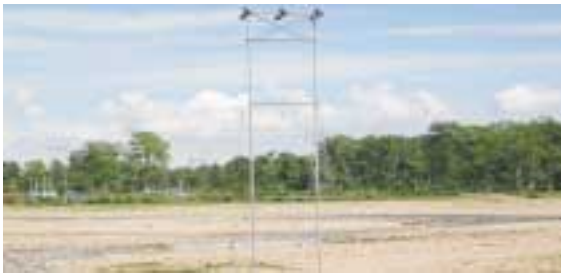
33 kV double pole structure at Khutia River crossing (213 m span)
