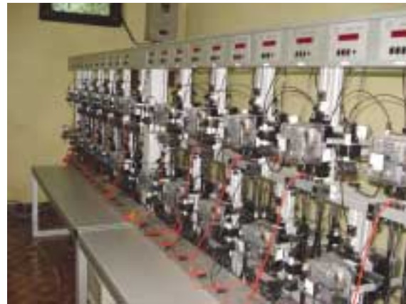
Meter Test Bench installed by REDSRP at NEA Hetauda
